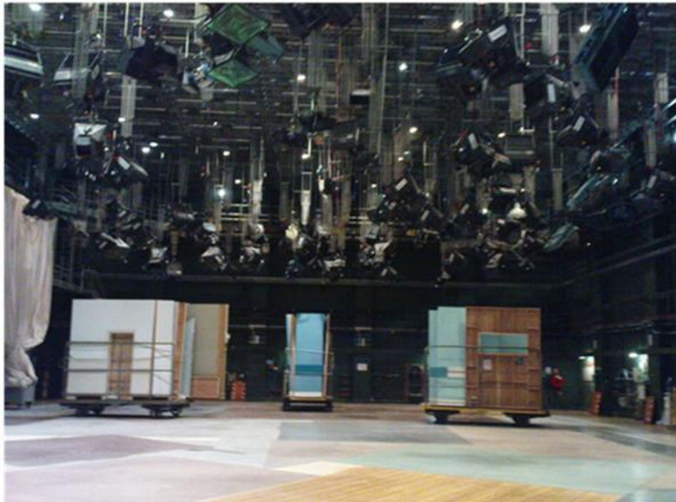
Figure 5.4: General view of Studio D
