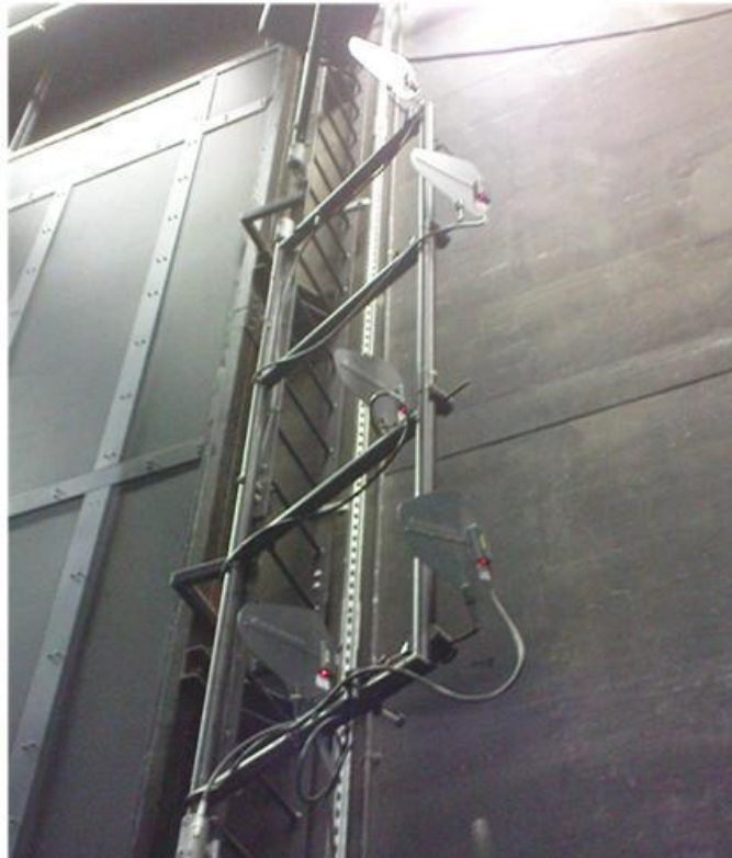
Figure 3.1: Showing microphone receive antennas in wings of Olivier stage
